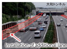
Installation of additional lane
