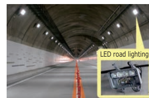
Install LED road lighting
